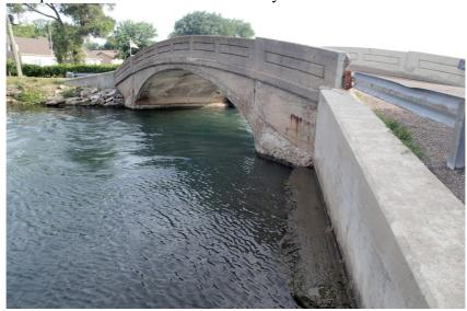
Work on the structure included the excavation of damaged material from the abutment faces, rebuilding the face with concrete material, and backfilling any voids that existed.
